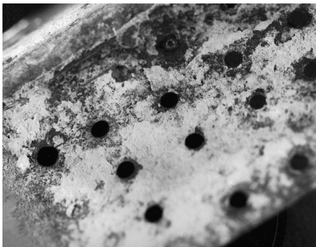
Figure 3-23. Aluminum Surface Corrosion Products
